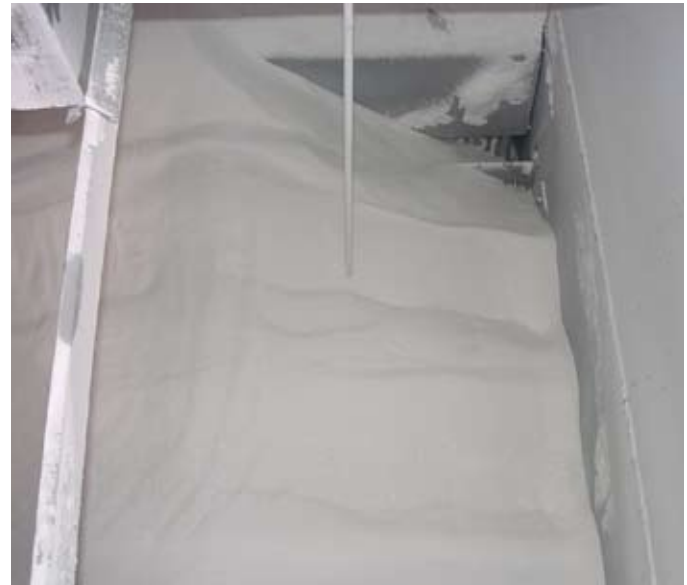
SUGAR LEVEL INSIDE COOLER INLET HOPPER
